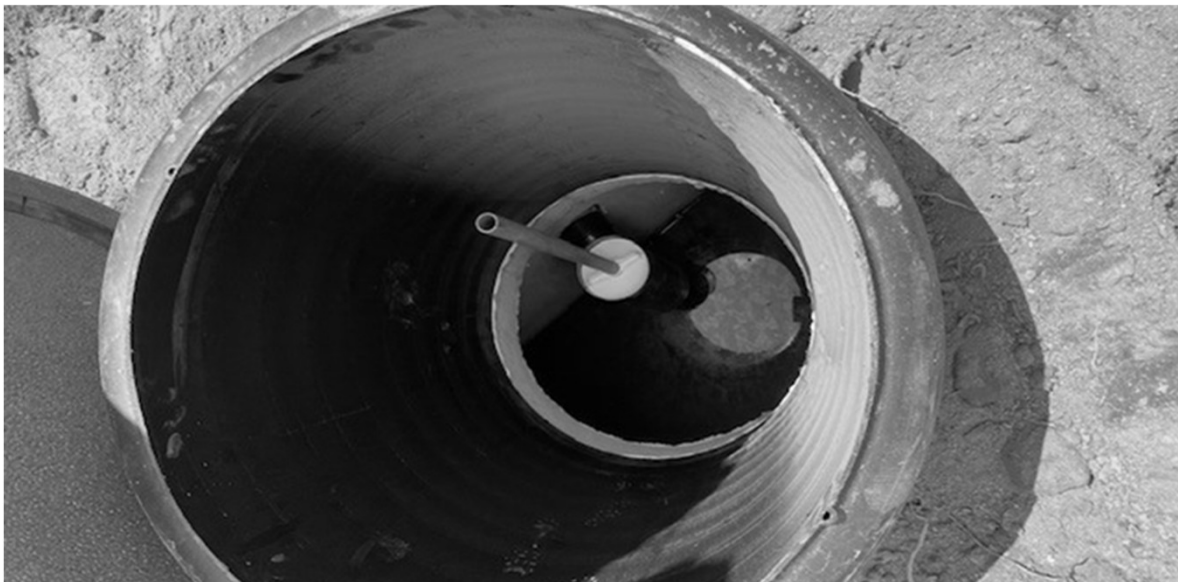
6" PVC Polylock PL 250 outlet baffle filter cartridge with cartridge. Handle attached for removal.
