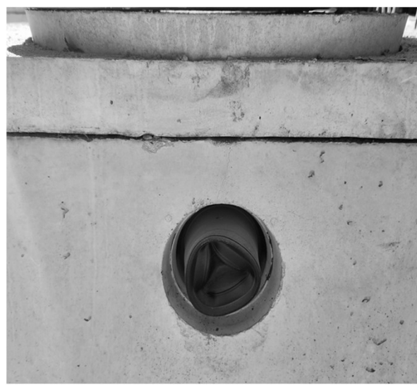
Outlet opening with mechanical seal 3" below inlet elevation
