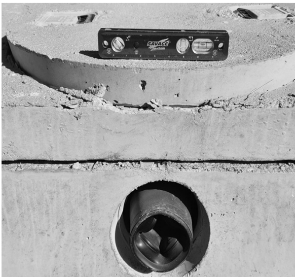
Inlet opening with mechanical rubber seal
