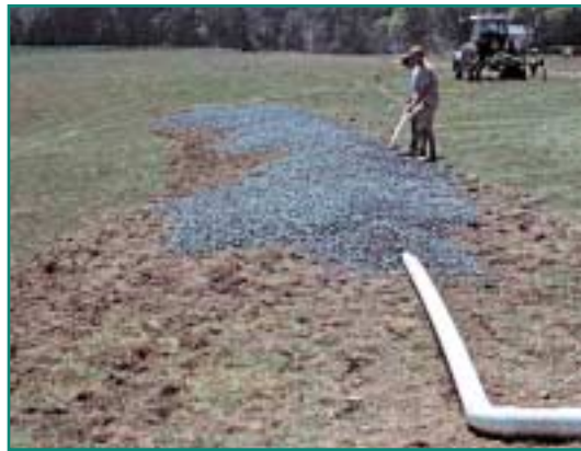
At-grade bed for wetland overflow
