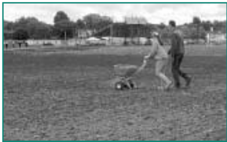
▲ 13. Seed being broadcast over the tubing areas.
