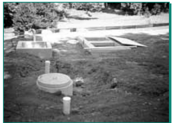
Septic, rock, and sand filter tanks
