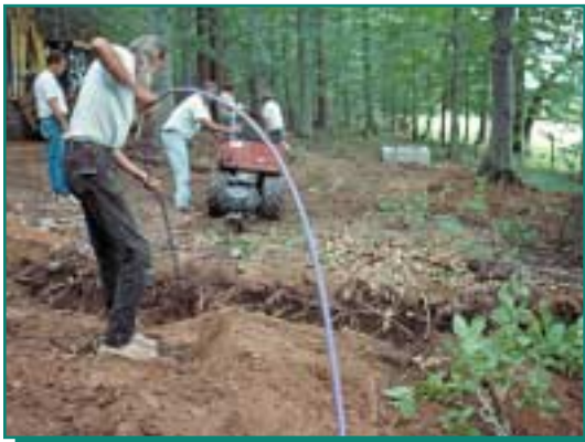
Drip tube installation
