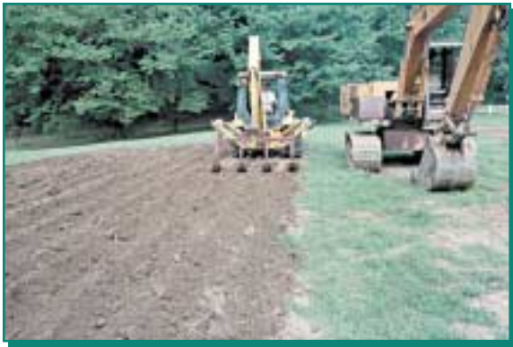
Placement of gravel on at-grade beds
